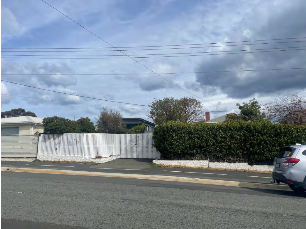
Image 1: 7 Talune Street, site frontage, northern elevation
