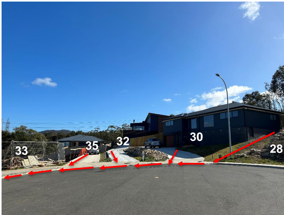
Figure 6: Property accesses for 35, 32 & 30 Belmont Court, red arrows show direction of fall
