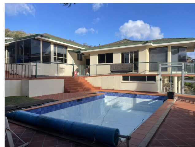
EXISTING POOL AREA AND ASSOCIATED TERRACES
