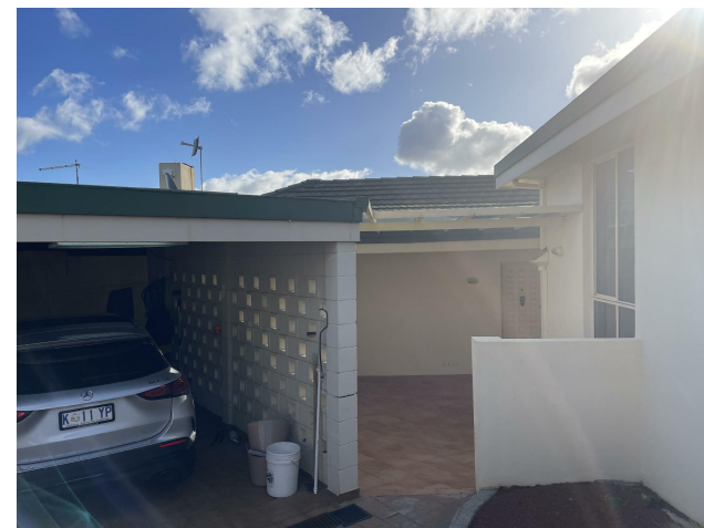
EXISTING CARPORT & ENTRY
