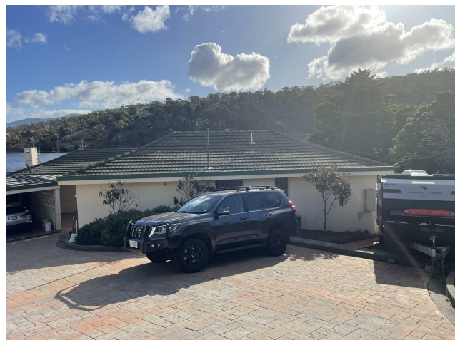
EXISTING FRONT (SE) FACADE
