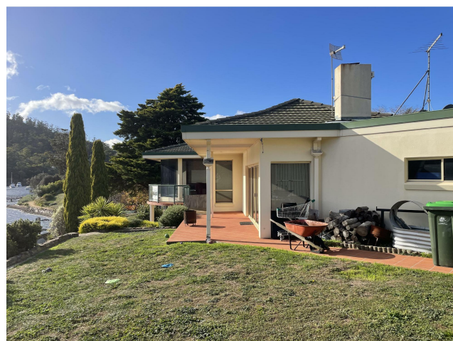
EXISTING SIDE (SW) FACADE
