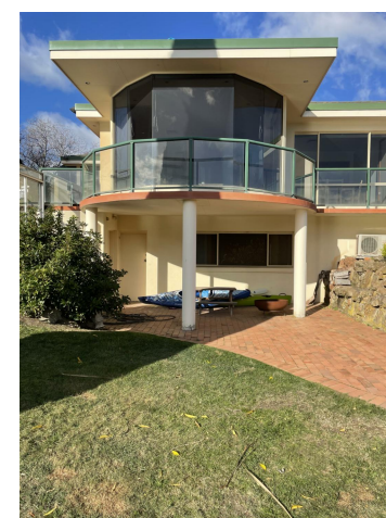
EXISTING REAR (NW) FACADE
