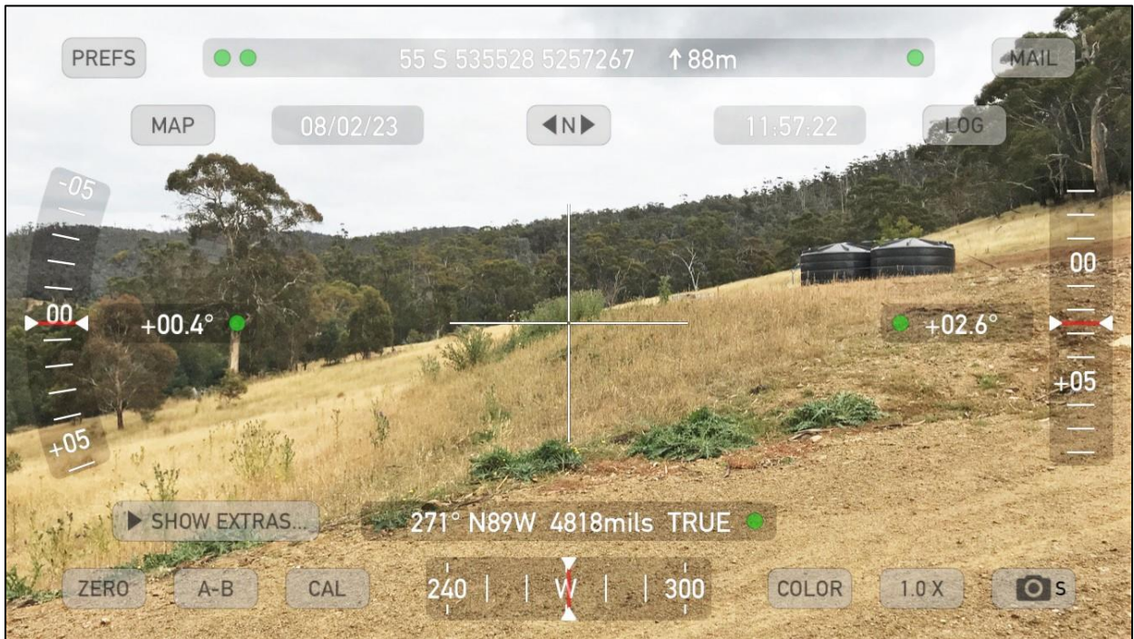
Photo 8 – Fill at the western end of the development site
