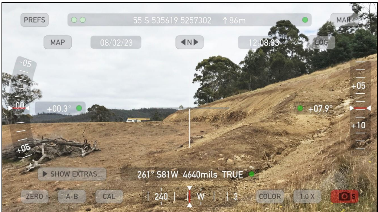
Photo 12 – Cut-and-fill at the eastern end of the development site, with proposed house site at central left
