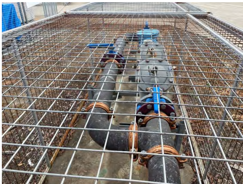
Figure 6 Meter Assembly
