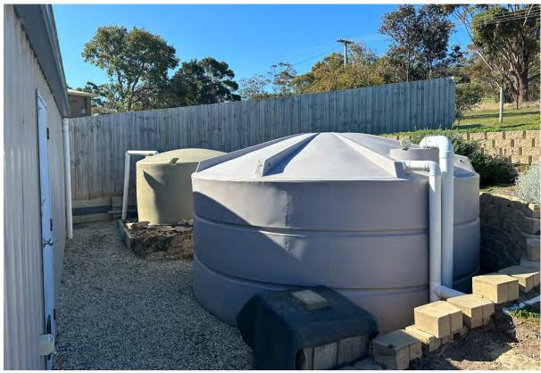
Photo 12: Field photo taken showing existing static water supply (for domestic supply) on proposed lot 2.
