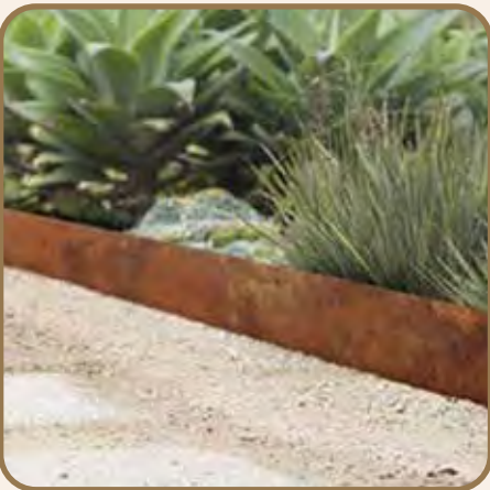
Back of footpath - corten steel
