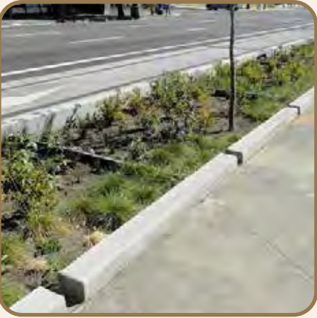
Street edge - split concrete kerb
