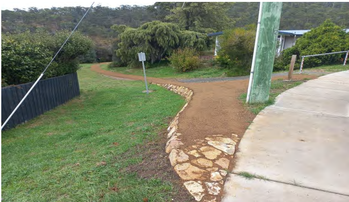
Figure 1 – Red gravel link track with dry stone edging at Granville Avenue
