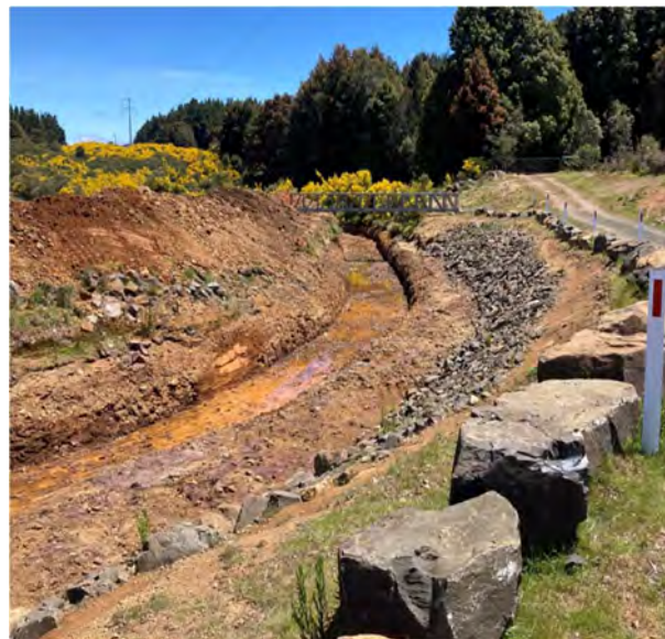
Waratah Dam – Dam safety improvements (spillway deepening, looking downstream)
