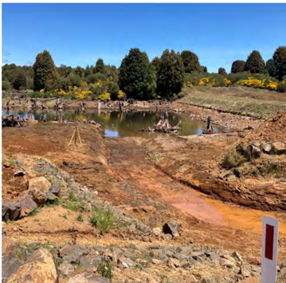
Waratah Dam – Dam safety improvements (spillway deepening, looking upstream)
