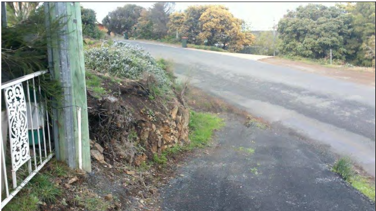
Photo 2: The view from the Otago Bay Road access towards Otago Bay Road demonstrating the safe intersecting sight distance deficiency to the south.
