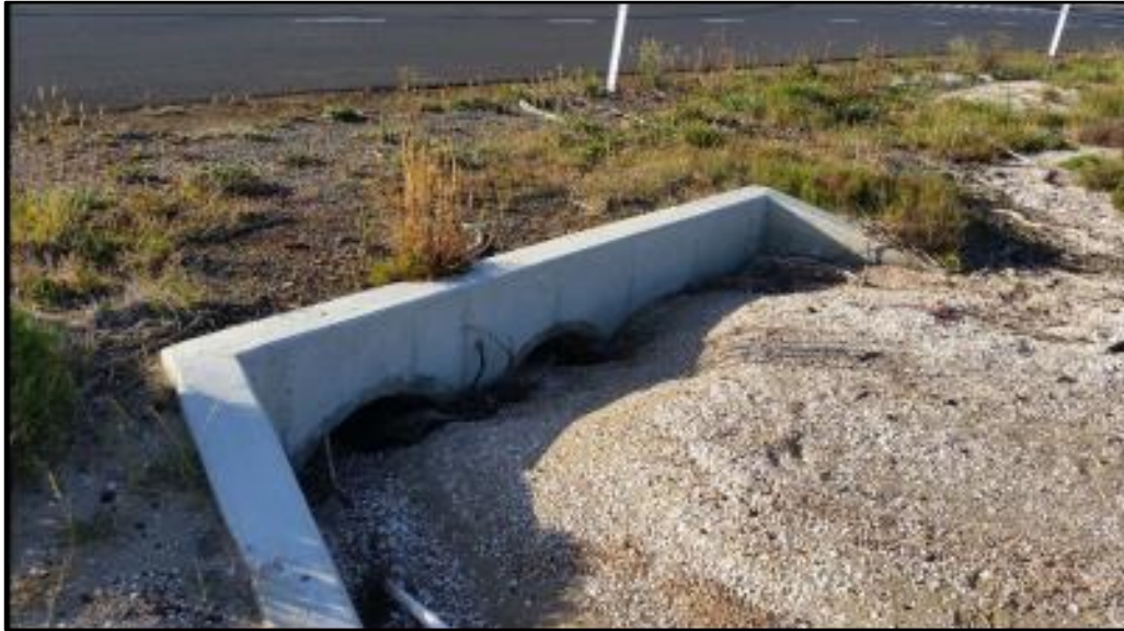
Figure 2: Blocked culvert (from DEP 2017)
