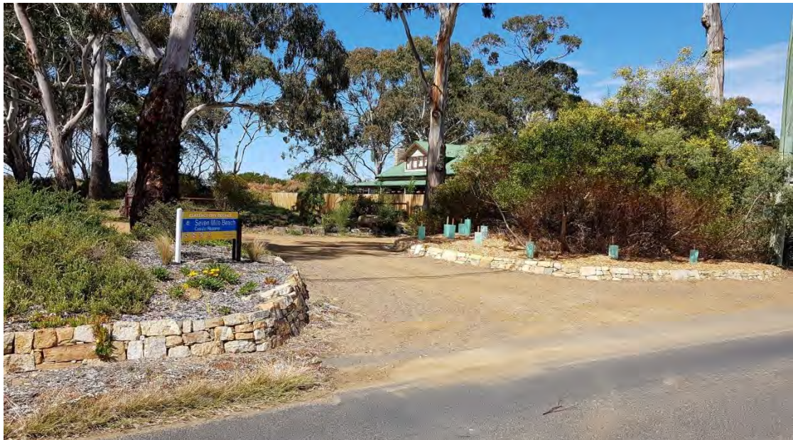
Figure 8 – Additional mudstone retaining wall (right) at Entrance to Seven Mile Beach Coastal Reserve from Sunways Avenue.
