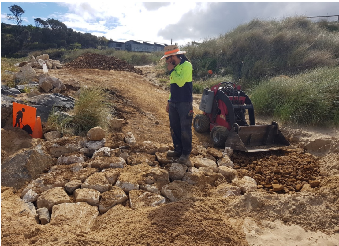
Image showing Rock Paving Installation at base of Water Access Ramp at Clifton Beach
