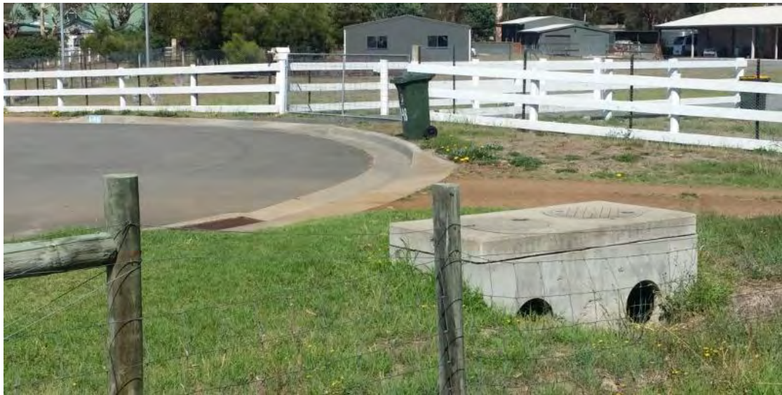
Figure 3-4 - Existing Culvert inlet from wetlands at Balook Street. Start of NT1
