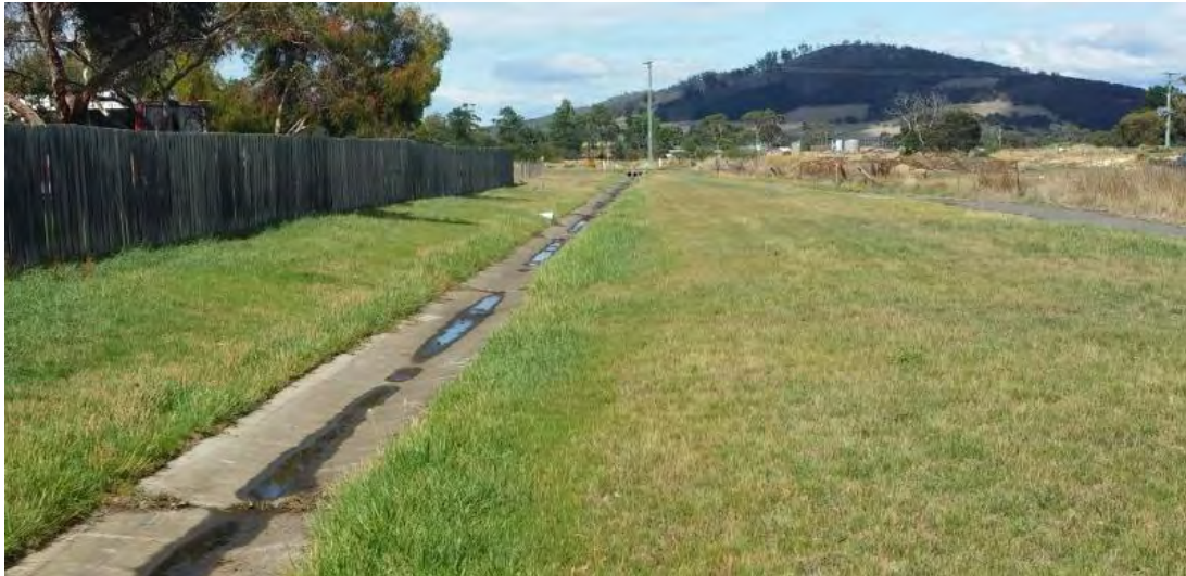
Figure 3-7 - Existing concrete lined open drain, NT1.
