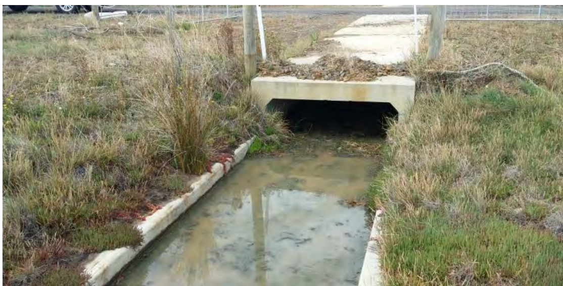
Figure 3-3 - Existing 1500x500 box culvert at CH.130 on NT2
