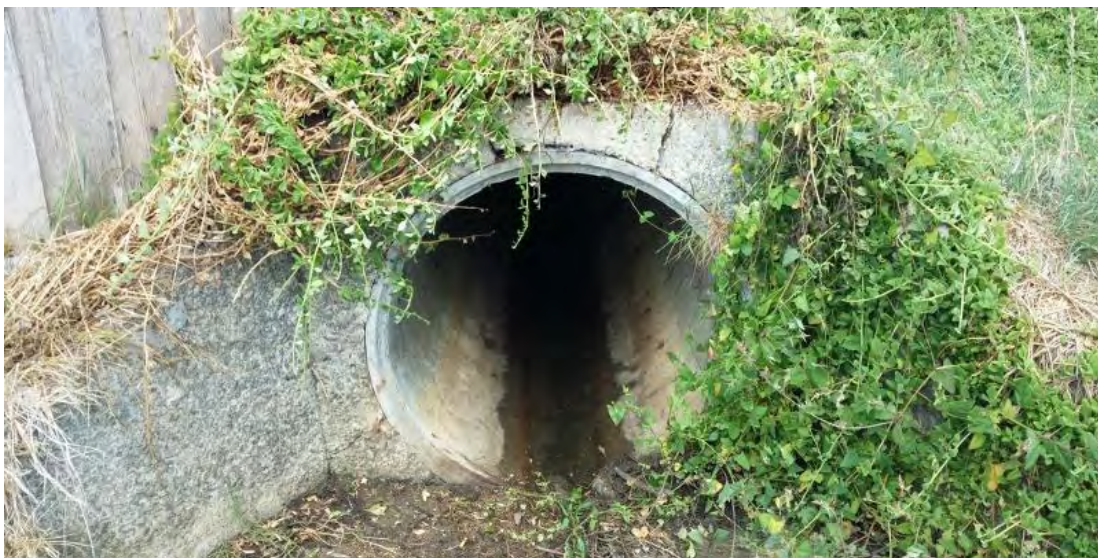
Figure 3-8 - Existing DN900 culvert at 12 North Terrace
