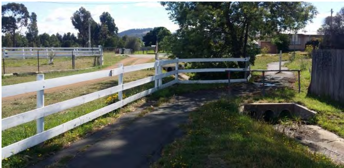
Figure 3-5 - Existing 3 x DN375 culverts under Balook Street
