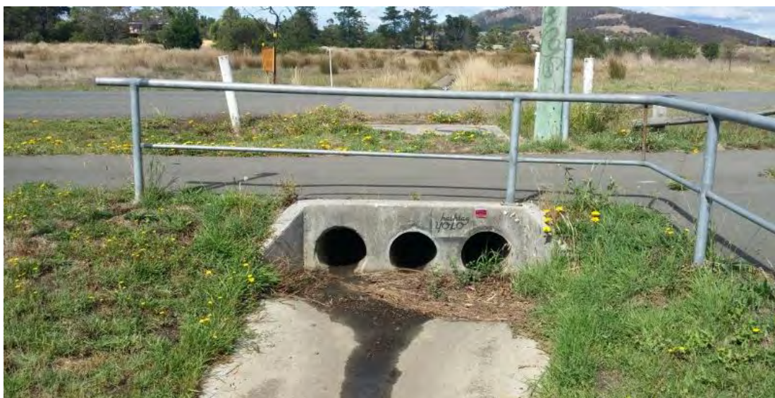
Figure 3-6 - Existing 3 x DN375 culverts under Mannata Street
