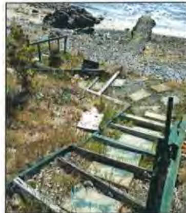
Plate 41 – Example of private steps to beach that have become unsafe due to lack of maintenance
