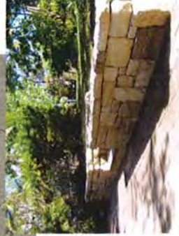
SANDSTONE RETAINING WALLS IN GARDEN.
